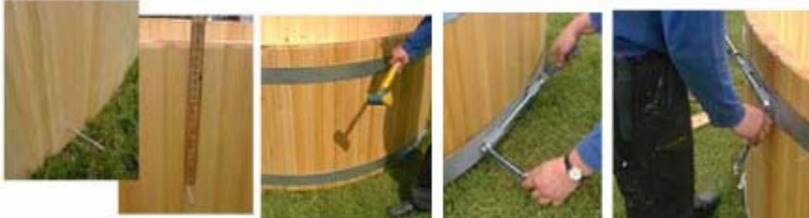
Note: During the tensioning you will hear the wood creaking. Do not worry about this, the staves are positioning themselves. The tensioning screws are subjected to a great deal of force. Ensure that there is about the same amount of thread on both sides.
