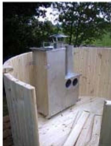
Mark and then drill 4 stud screws into the wall of the tub. This can be done easily by clamping the stud screws in the drill head. Now fix the stove with the wing nuts on the inside of the staves.
